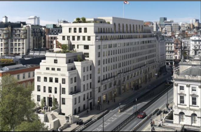
Brettenham House Main Works commenced Summer 2024
